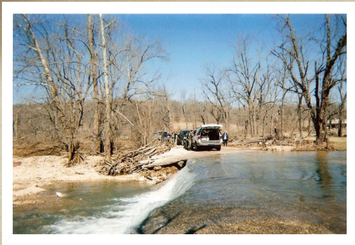
The Bridge and Creek
